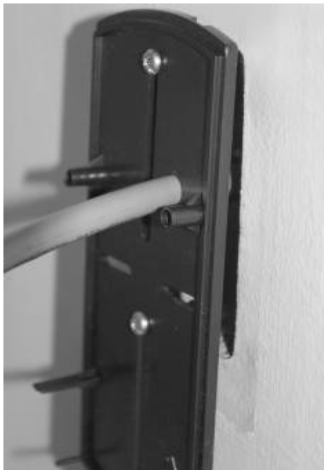
Figure 9> Installing back plate to the wall
